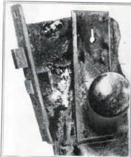
After the fire, the lock on the door that barred the way to escape was found. The bolt was still out.
